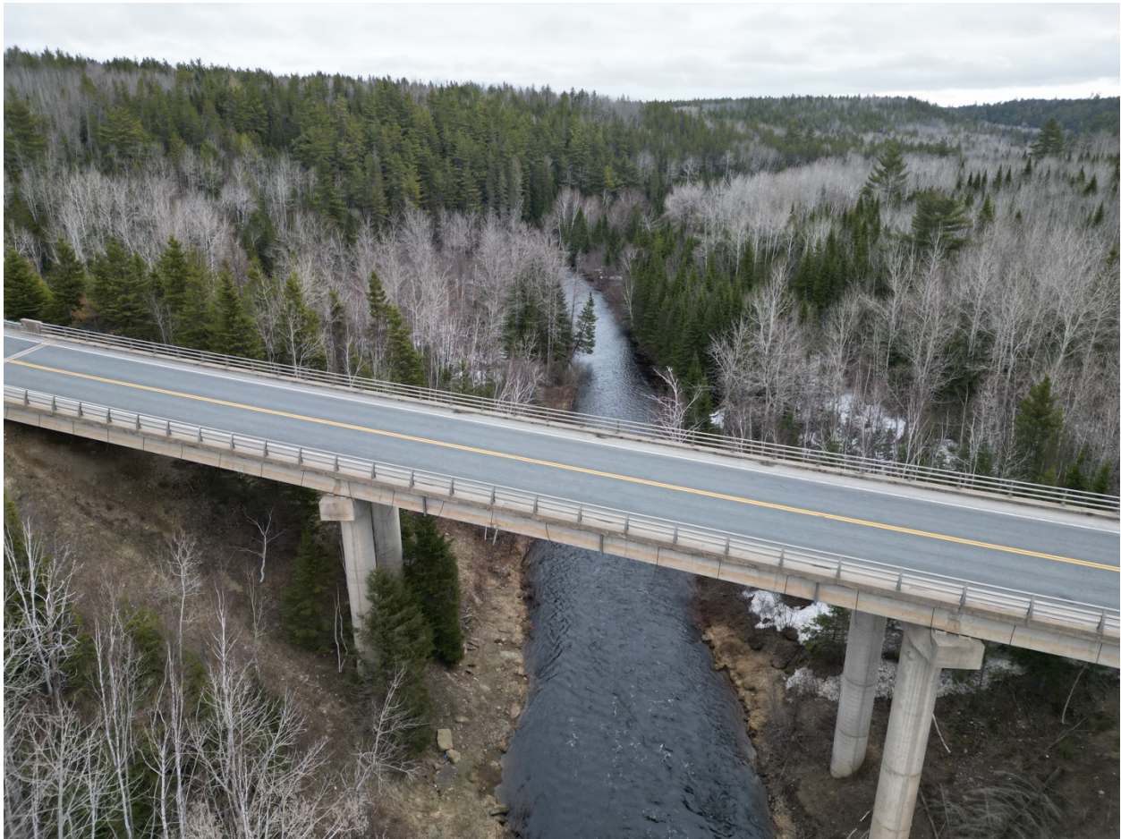
Figure 20 Looking downstream at Tabusintac River above Highway 8
